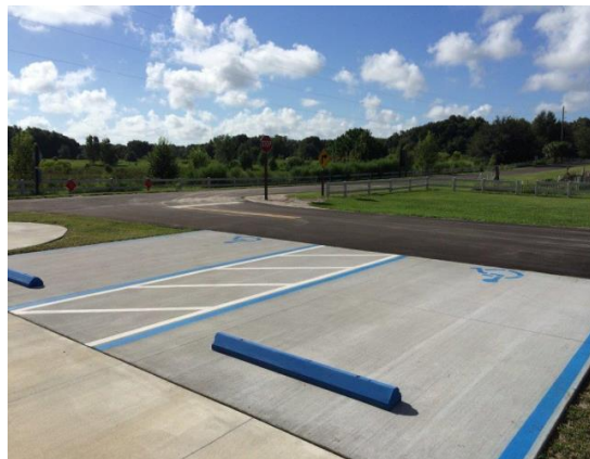
ADA parking improvements at P.E.A.R Park completed in FY 2018
