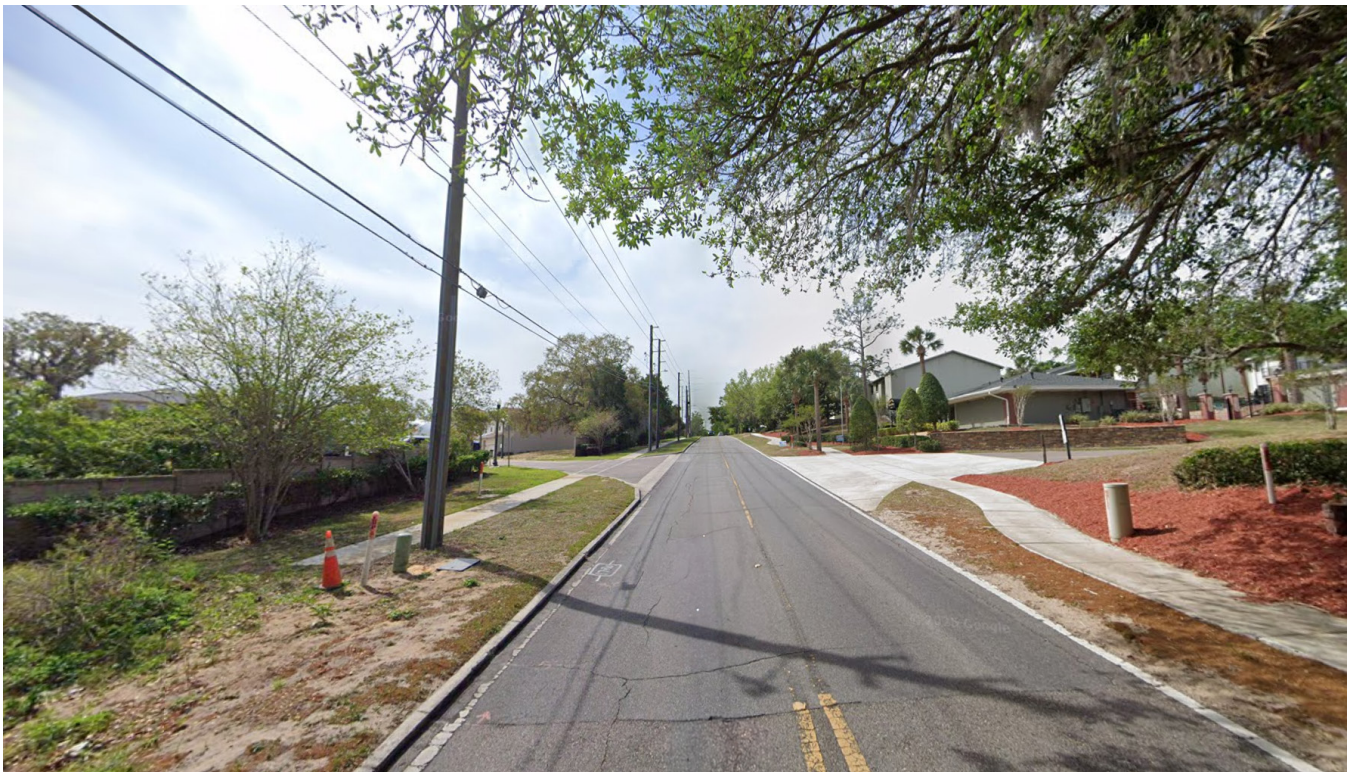
Figure 7. Picture of S Grand Highway between Pitt St and E Hwy 50 in Clermont
