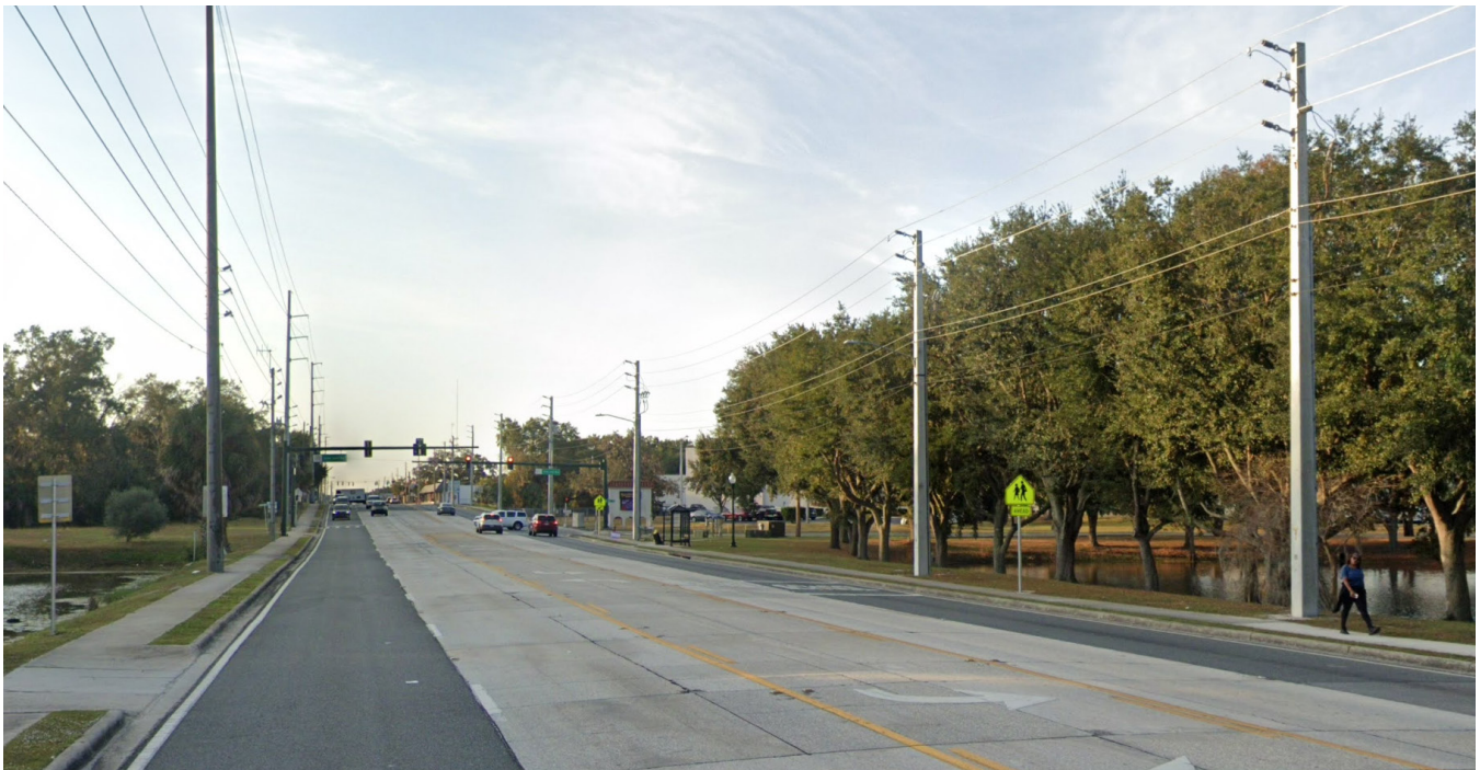
Figure 5. Picture of N 14 th Street between Dixie Avenue and Main Street in Leesburg
