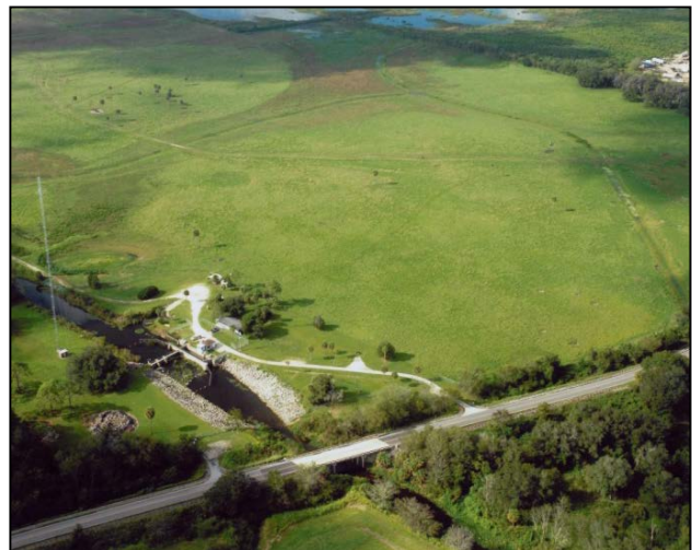
NuRF Site, October 4, 2007, pre-construction
