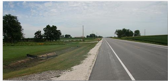
A paved shoulder is often the bicycle facility associated with a rural road.
