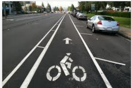
A buffered bike adds additional separation between bicyclists and vehicles.
