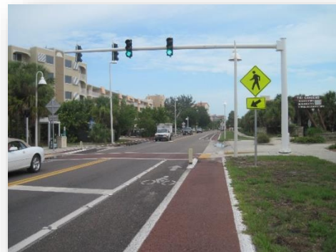
A pedestrian hybrid beacon helps stop traffic when actuated so a pedestrian can safely cross
