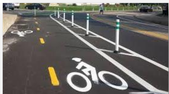
A separated lane adds an additional physical separate between bicyclists and vehicles.
