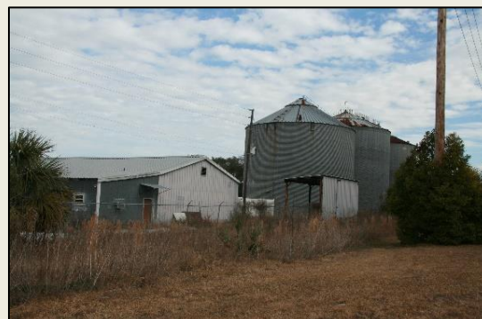
"Abandoned commercial developments."
