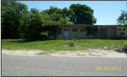
"Abandoned residential unit."
